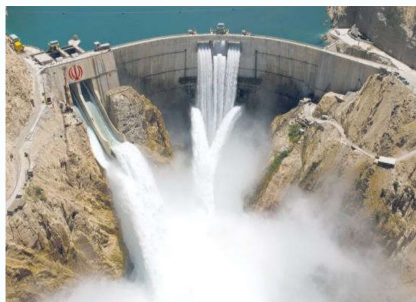
Karun III 205 m high concrete arch dam, service, auxiliary and emergency spillways
