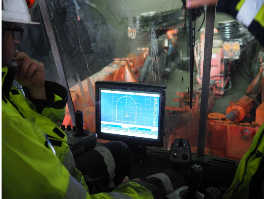
Figure 3. Borehole contours based on the BIM-model shown on a display in a tunnel rig. Example from the new Mjåvatn dam and water tunnel in Norway.
