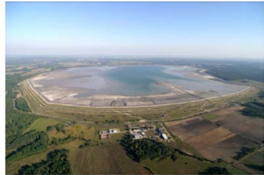
Figure 2. Tailings disposal, aerial view.
